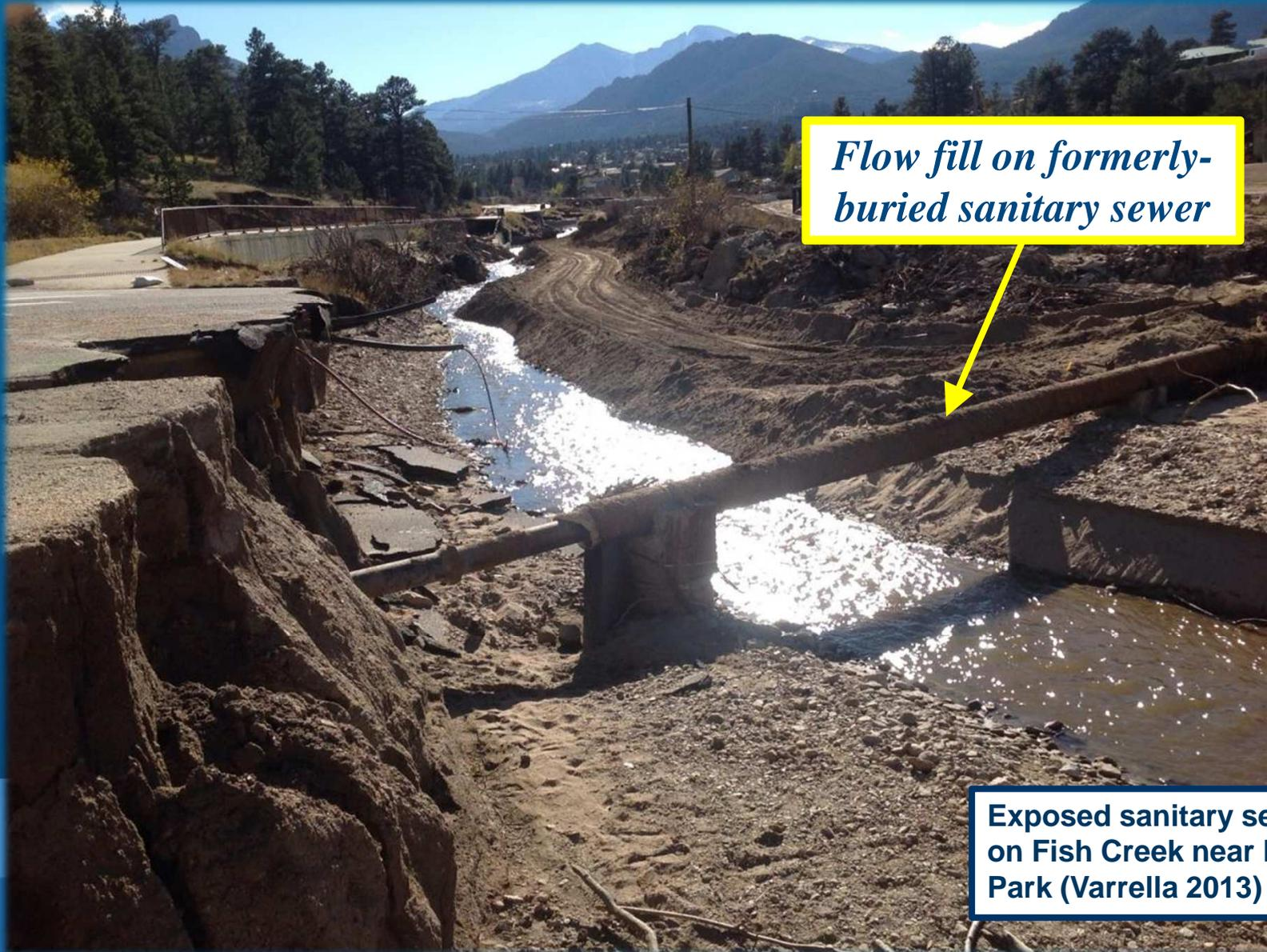
*Flow fill on formerly-buried sanitary sewer*
