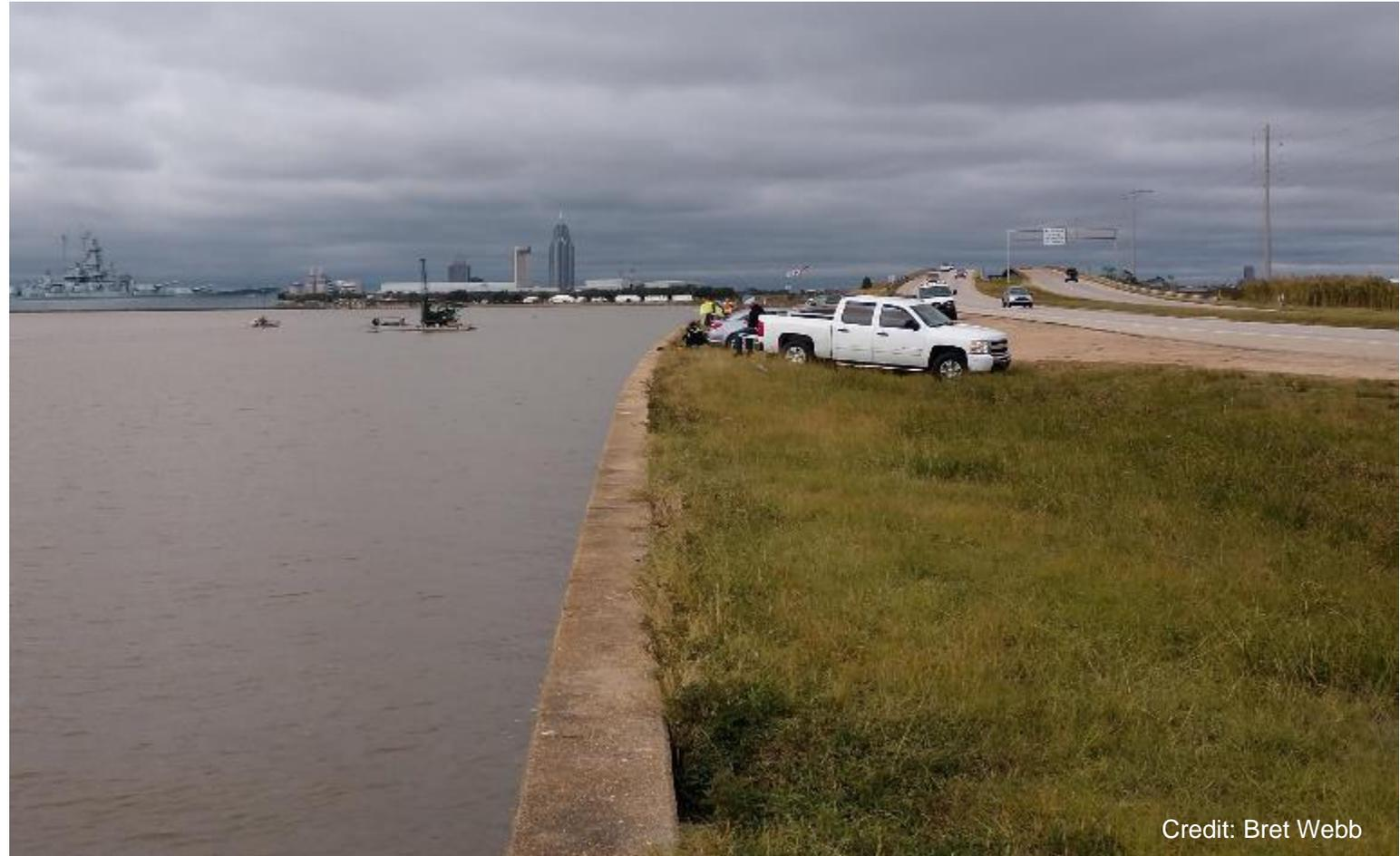
An existing concrete seawall serves as bank stabilization for the Mobile Bay causeway.
